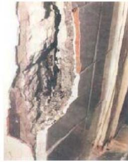
Main Reinforcement corrosion and spalling of concrete
